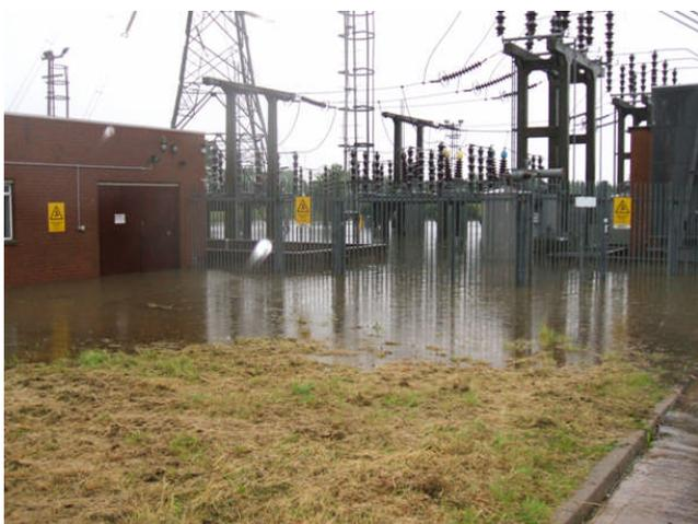
Castle Meads substation in Gloucester flooded and was switched off to protect the equipment. Supplies to 47,000 customers were lost initially and were progressively restored within 20 hours.
